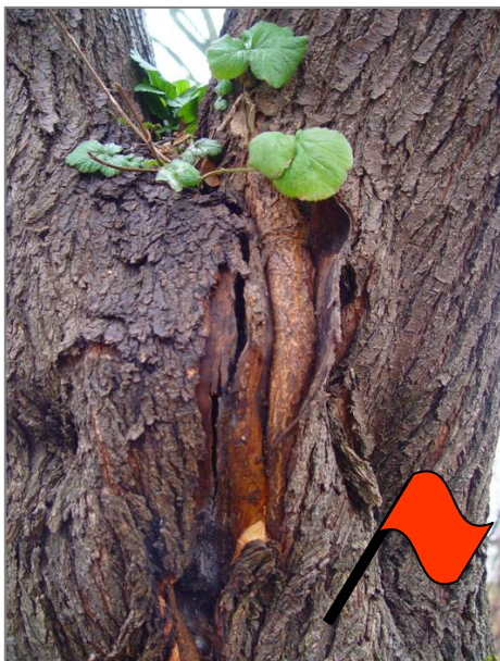
Crack in branch union, Horse Chestnut
