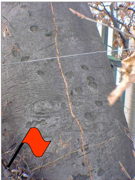
Fresh crack through the stem
