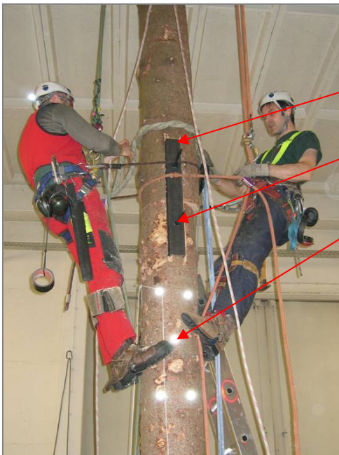
Attachment of a new top section
