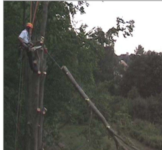
Stage 3 - lowering a tree top, final phase, interval 0.2 sec (drop no. 1)
